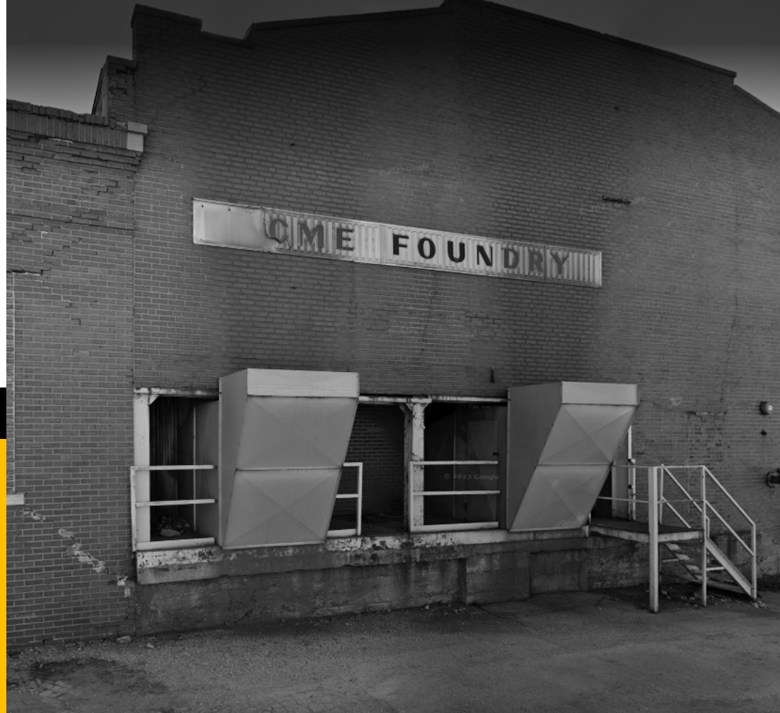
Acme Foundry Building Source: Google Maps
